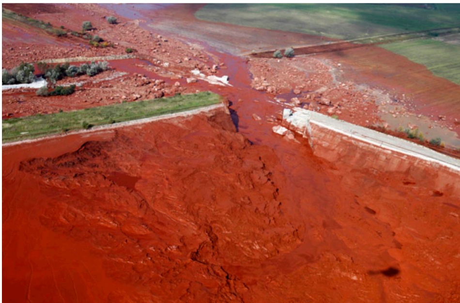
Bild 2: Dammbrottet i damm nr 10 vid aluminiumfabriken Magyar Aluminium Zrt i Ajka. Foto: Ministry of Public Administration and Justice, Ministry for Government Communication [Public domain], via Wikimedia Commons.
